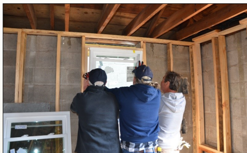
Construction Ministry installation of windows for Family Promise homes located on Cumming Street
